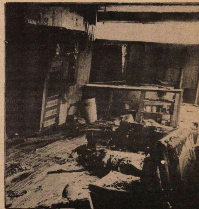
Burned remains of Community Center offices.
