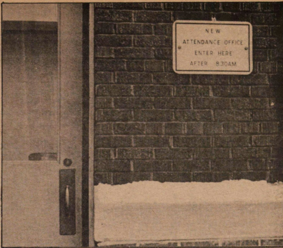
Everyone & anyone who enters Pontiac Central comes through an administration office. All other doors are locked with two guards keeping watch.
